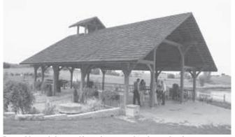
Post and beam shelter provides a place to go when the weather does not cooperate. The Nortons built it from scratch, using timbers from old barns and grain elevators.
