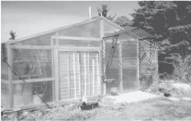
Harry Benjamin assembled this heavy-duty greenhouse in his shop during the winter, welding together salvaged material to build it. Structure is anchored to a concrete floor.
