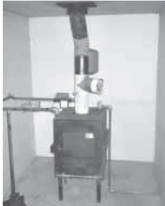
Measuring 20 in. wide, 24 in. deep, and 25 in. high, boiler handles 18-in. logs.
