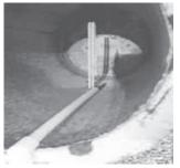
Heater's original element was replaced with a 4.500-watt element. Thermostat's bulb sensor is protected by a section of PVC pipe added inside the tank.
