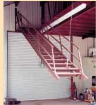
Drop-down stairway is 17 ft. long and has 15 steps. Cable disconnects once ladder is down.
