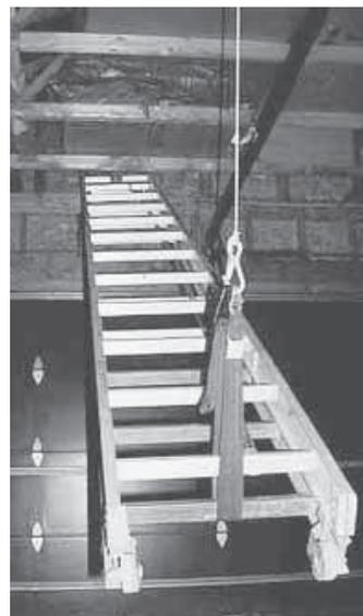
Richard Bergman came up with a pulley and counterweight system that lets him store his 20-ft. extension ladder out of the way above his overhead garage door. Ladder is held up by a counterweight that goes up and down easily.
