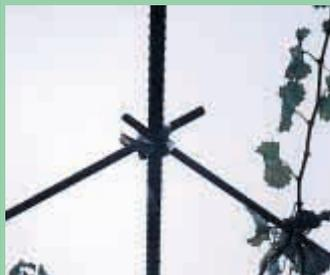
Water hose clamps hold rebar structure together.
