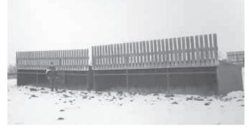
Windbreak extends about 3 ft. above shelter's roof to keep wind from blowing down right in front of shelter.
