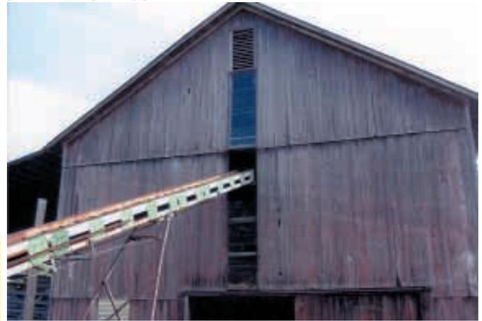
Barnosky removed vertical wood siding to make an opening about 32 in. wide from top to bottom of his barn. He then installed a line of removable windows in opening.
