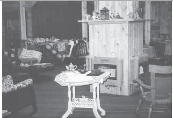
Four heaters mounted on central support heat the large structure.
