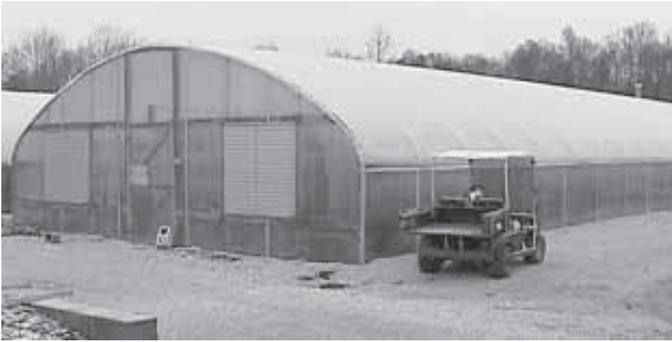
One of the greenhouses that Cretella built out of 1 3/8-in. dia. galvanized tubing. Note the 4-ft. straight sidewalls.
