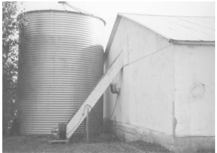
Engler put a 2,400-bu. bin at the end of his hog barn. To get hot air from the barn attic to the bin, he made a 16-in. sq. duct from plywood and connected it to the intake side of an aeration fan that he mounted inside the bin.
