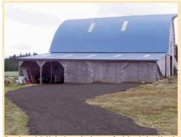
Ground-up asphalt shingles give you the advantages of asphalt paving but without the cost. An Oregon company came up with the idea.
