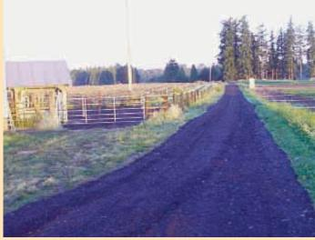
Recycled shingles can be used to pave farm driveways and feedlots, as well as alleys and walkways around buildings and livestock pens.
