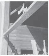
The two doors meet inside the bracket, which keeps the doors rigid so they can't blow either in or out.
