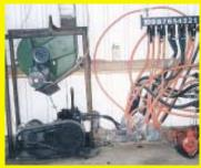
Blower, hydraulic pump, temperature controls, water pumps and reservoir are located in the building next to furnace.
