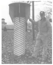
Submarine "snorkel" sticks out of ground about 150 ft. from house. Snorkel connects to a 12-in. dia. plastic pipe that runs underground to house. Outside air is drawn through pipe by a fan during summer to provide "free" air conditioning.
