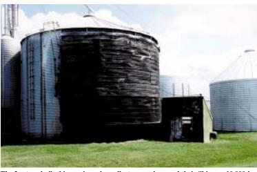
The Lortons built this passive solar collector panel around their Shivvers 10,000-bu. grain drying bin. Sheets of tin, painted black, run from under eave down to the ground.
