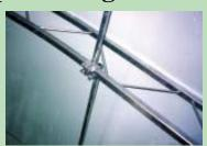
Trusses are made from square tubing, webbed together with solid steel bars.
