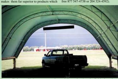
Stream Shelters welds its trusses together and then galvanizes the finished product. "That makes them far superior to other products which are galvanized first and then welded together. We treat the entire truss, including the welds," notes Darryl.
