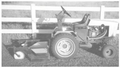
Ernest Bueckert turned a Case 444 hydrostatic-drive garden tractor into a zero-turn mower by reversing it and mounting a 54-in. deck on front.
