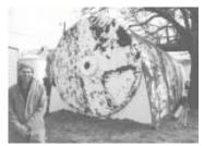
Ballinger left the bottom in the end tank to form a back wall.
