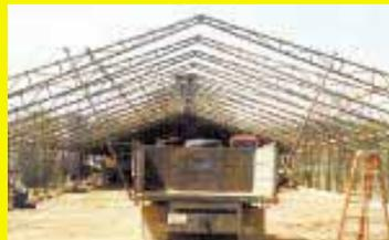
the sides of our Ford truck to take down the trusses. They bolt to the frame and support the truss while we disconnect it at the ends. They simply hook over the
