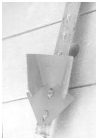
**As soon as post starts to move up, wings on the top half of the anchor flatten out to keep post from going up any farther.**
