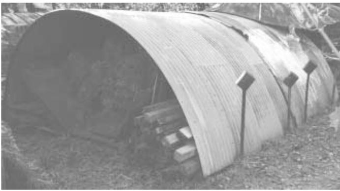
Low-cost shed was made by placing two bin halves side by side on ground and using steel posts to keep the sides from spreading out.
