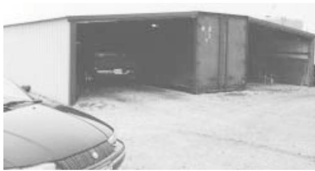
An 8-ft. high shipping container serves as the center support for Robert Dunton’s 40 by 40-ft. shed. A 16-ft. wide metal roof extends out each side from top of container.
