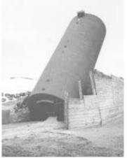
The 30-ft. long fuel tank mounts at a 60-degree angle next to Sylla's wooden-walled bunker silo.
