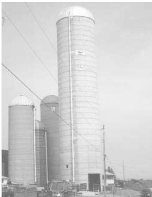
Poured cement silo stands 132 ft. tall not counting the 15-ft. dome on top. Note drive-through alley.
