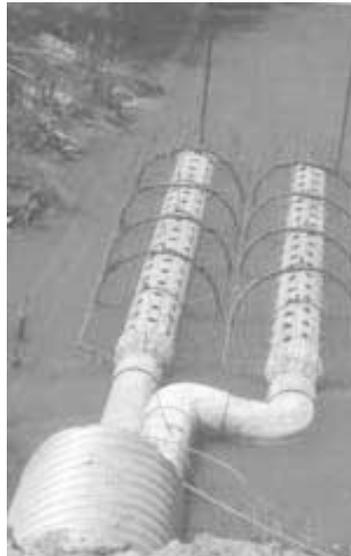
Beaver Pond Leveler creates a leak in a pond that can't be plugged. It consists of pvc pipe with holes in it suspended inside a wire cage. The large number of holes in the pipe spreads out the flow of water to keep the current to a minimum.
