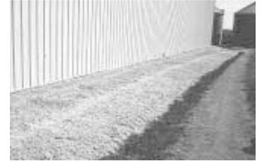
A 2-in. layer of loose rocks, laid on top of a layer of plastic, stops rodents from tunneling into building.
