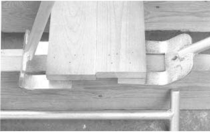
"Gerry Bar" has a pair of steel prongs that lift from underneath with minimal damage.
