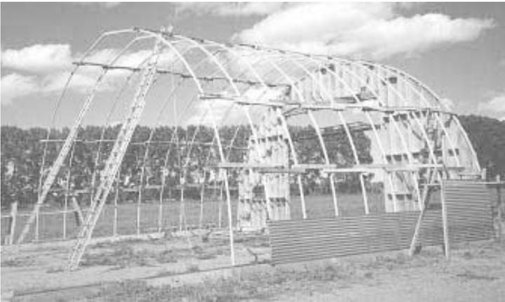
Lightweight tubing, commonly used in oil fields, was used for the framework.
