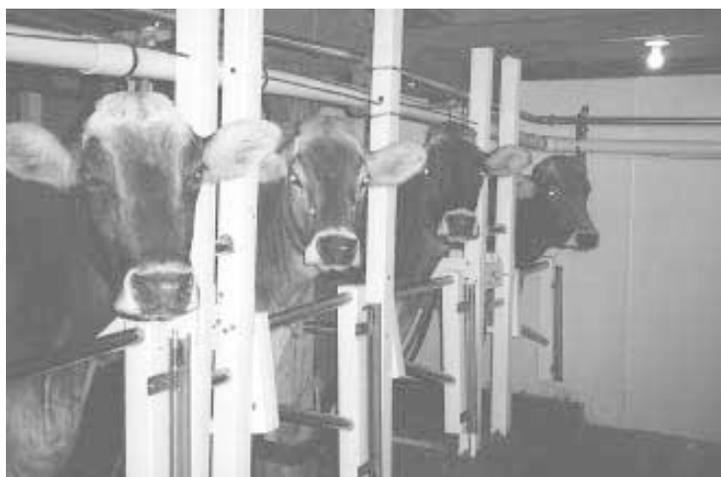
“It’ll never rot or rust and it cleans up like new,” says Gary Lisowe about the 4-unit milking parlor he built out of recycled “plastic lumber” and stainless steel pipe.
