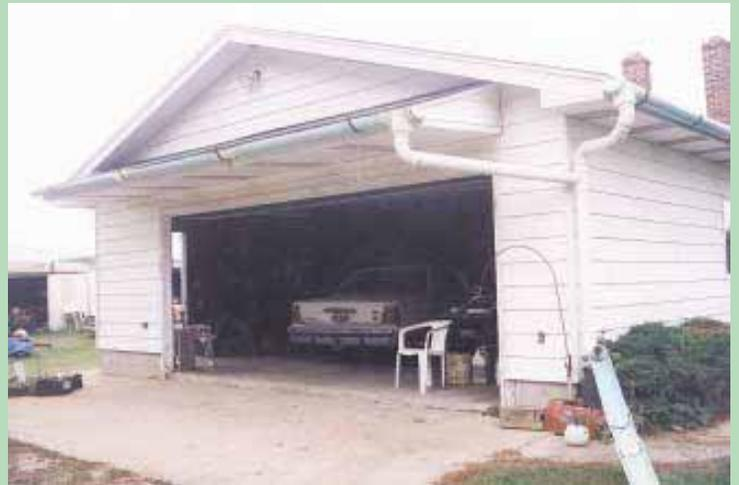
Kaiser used lengths of 6-in. dia., 1/4-in. thick plastic sewer pipe to make eave troughs and down spouts, cutting sections of pipe in half lengthwise and bolting them together.
