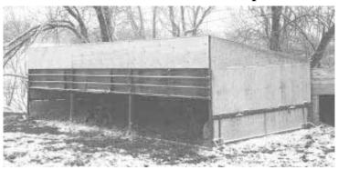
Shelter measures 7 ft. high in front and 5 ft. high in back, with a frame built of 2 7/8-in. dia. oilfield pipe covered with plywood. The front part is equipped with removable horizontal bars that can be removed, bottom to top, as calves grow.
