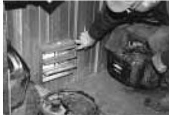
A 1/2 hp squirrel cage fan blows air out of the collector and into the building through five 1-ft. sq. louvered vents located along base of wall (above). Solar collector panel covers entire south wall of the Lorton's 16 by 50-ft. combination machine shed and shop.
