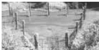
"Beaver Deceiver" consists of wooden fence posts in a trapezoidal configuration covered with mesh wire.
