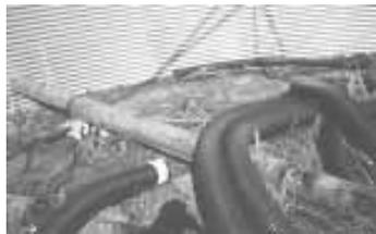
Floor consists of a layer of plastic on top of a gravel and clay base. A length of 12-in. dia. tile is placed on top of plastic in a circle about 6 in. from bin sides and also goes vertically to top center of bin. A fan blows air through tile to provide aeration. Photo was taken after bin was emptied.
