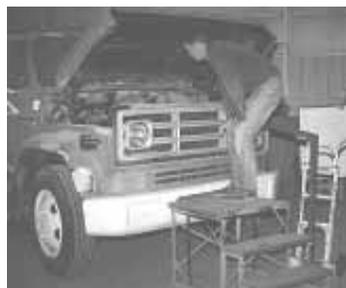
"A set of mobile home steps makes it easy for me to access truck engines. I use a 2-wheel hand cart to move the steps."
