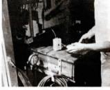
I had a close call at one time using a nongrounded drill so I came up with this portable grounding box for using tools away from the shop. Makes using 2-wire hand tools much safer. The box, which would normally mount on the wall, just plugs in between an extension cord and the drill. You can buy grounding boxes from electrical suppliers or at discount stores. (Roland Beckmeyer, Hoyleton, III.)
