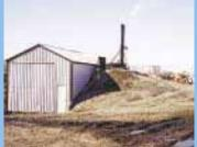
Furnace is buried in an earth berm next to a 16 by 32-ft. shed. The Klimacks burn about 40 5 by 6-ft. round bales of flax straw a month in the coldest weather.
