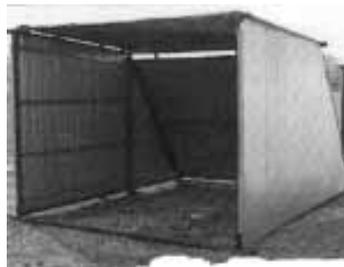
Livestock shelter consists of a 1 1/2-in. tube steel frame covered by corrugated metal.
