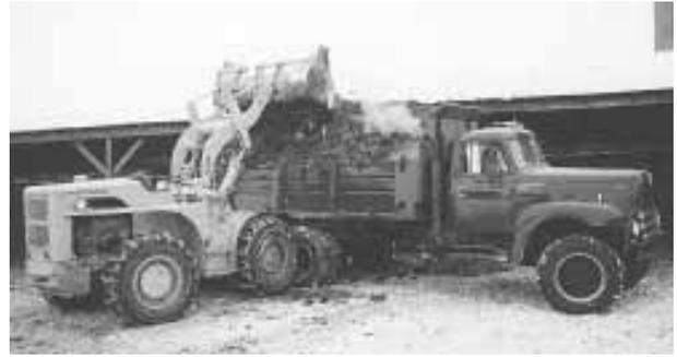
Used Farmhand manure spreader mounts on 1960's all-wheel-drive International tandem axle truck. Box is equipped with two rear beaters.
