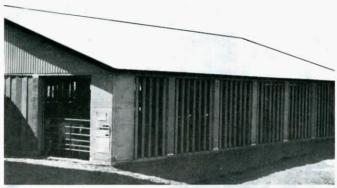
Vertical precast concrete louvers can be push-button controlled to "open the wall" or close it up tight.
